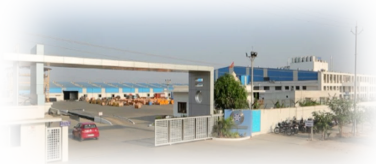
<< Cable plant at Khatalwada
