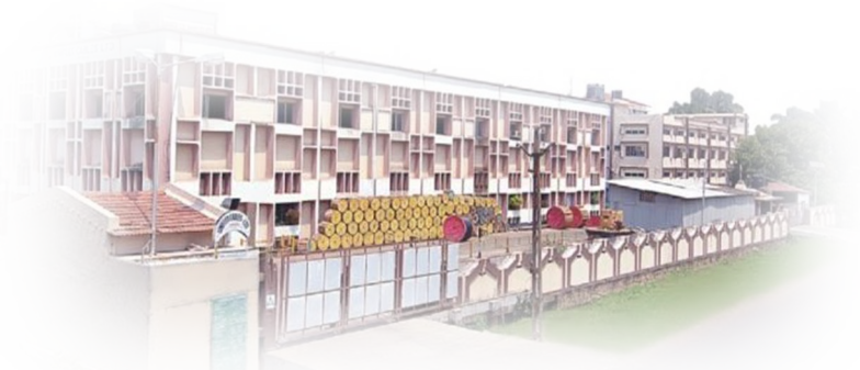
Cable plant at Umbergaon >>
