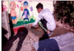
Civil Work at Anganwadi
