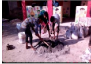
Civil Work at Anganwadi
